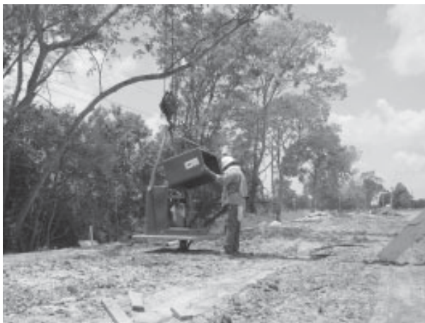
Fig. 5 Contractor feeding cable through compartment
