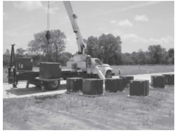
Fig. 2 Boom truck crane operator off-loading JSRP Transformer
