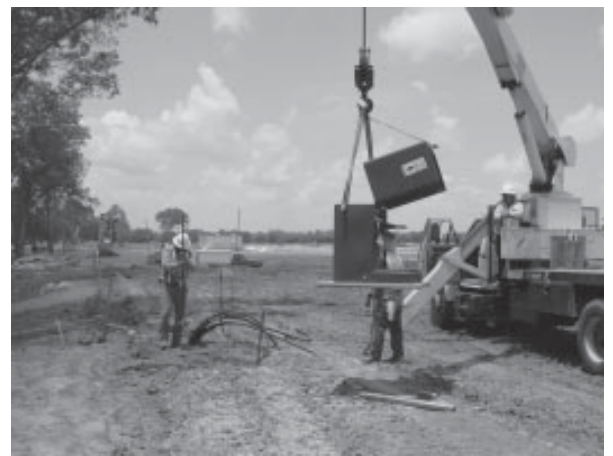
Fig. 4 JSRP Transformer descending to final installation site
