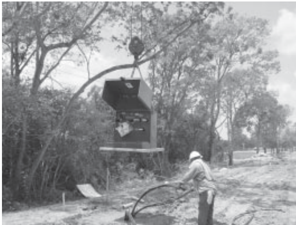
Fig. 3 Contractor setting up for installation
