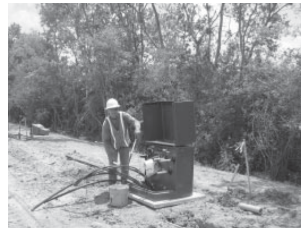
Fig. 6 Contractor completing installation of JSRP Transformer
